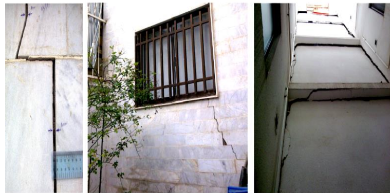
Adjacency damages (Marseh et al., 2013)
